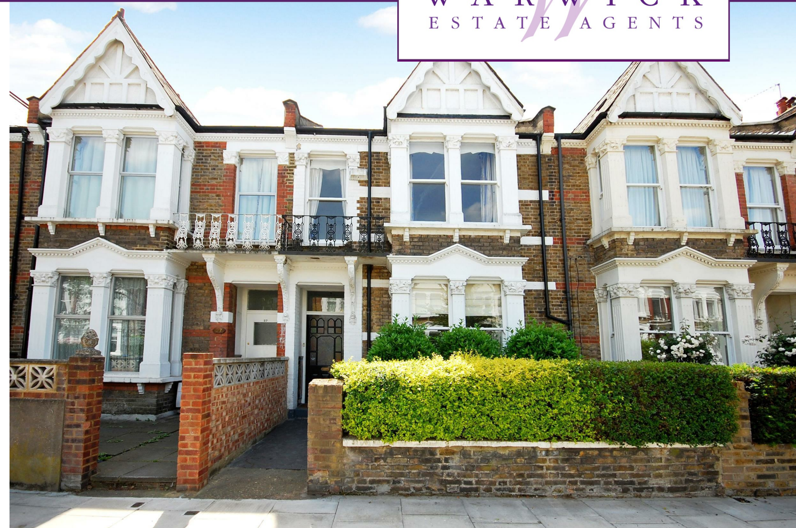
Kempe Road, Queens Park, NW6 6SP
